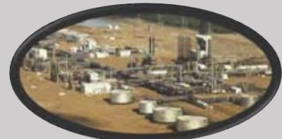
Thermal & Refinery Projects
